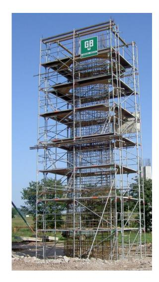
This upright for a railroad bridge is constructed of steel mesh and concrete. How do you think it would perform under mechanical load if:-
